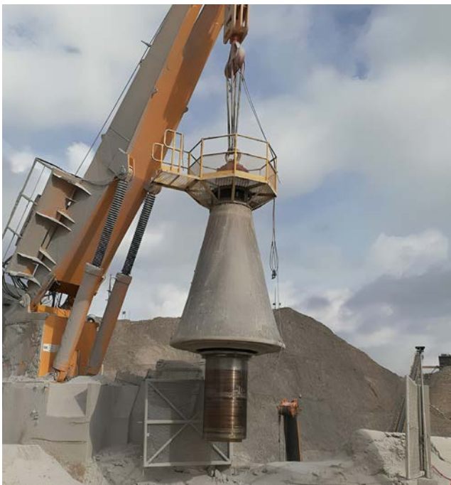
Figure 2. The crusher's 110 t mantle is extracted, exposing the damaged bushing.
